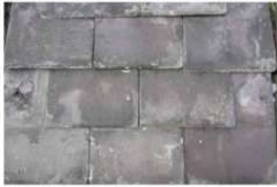
Example of: Slate Wall Shingles / Cladding (Photograph indicative) Roofing slate installed as rainscreen cladding on vertical external walls.
